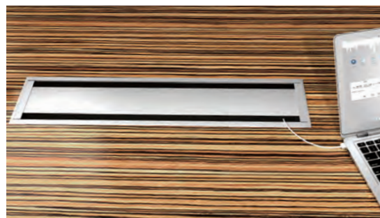
会议桌线盒，两侧都能打开走线 Open the wiring at both sides of the line box of conference table.
